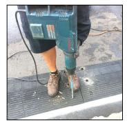
Step 5. Premark the drill bit to 8"deep either with tape or paint. Standing on first corner module and using a 9/16" drill (12" or 18" or longer) bit, drill through the existing module holes of the first row using the hammer drill, drill 9/16" diameter holes into the asphalt. The holes should be 8"to 9" deep in order to accommodate the standard 7" anchors. (if using 4" hardware, drill hole depth to 5" to 6"). 4" hardware best used for concrete or "snow belt" areas.
