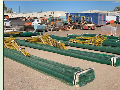
VIEW OF NEW 30 FT STEEL LIGHT POSTS
